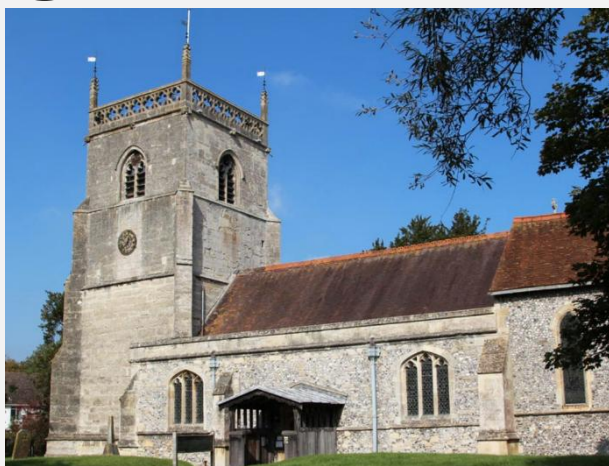
St. Michael's church, Blewbury. Lovely building.
